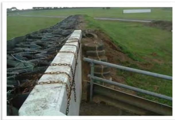
Image: Transition of concrete barrier into earth backed tyre wall. Note chaining of tyre wall stacks to each other and also linking the buffer system back to barrier.
